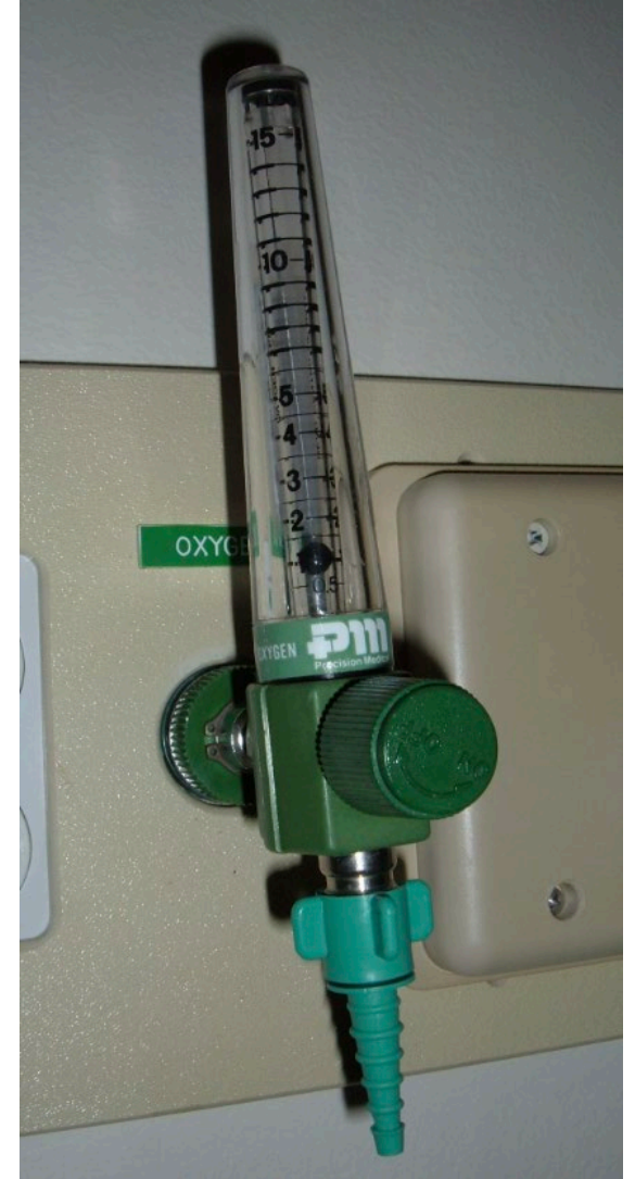
Wall mounted oxygen regulator valve
